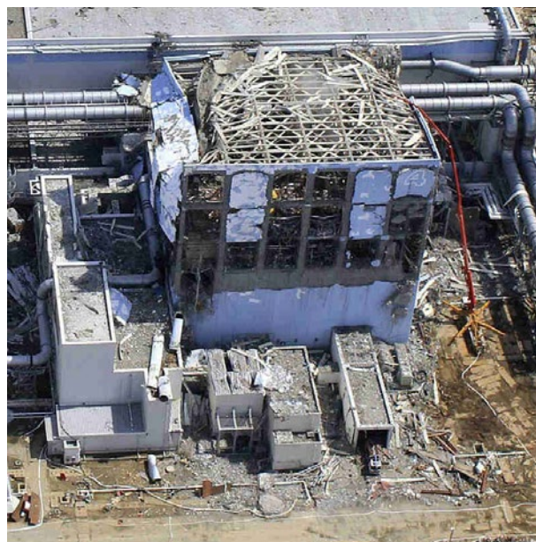
Figure 7: Damage to Fukushima Daiichi nuclear power plant's unit 4 reactor by explosions and fires caused by the earthquake and tsunami (Source: Air Photo Service)
